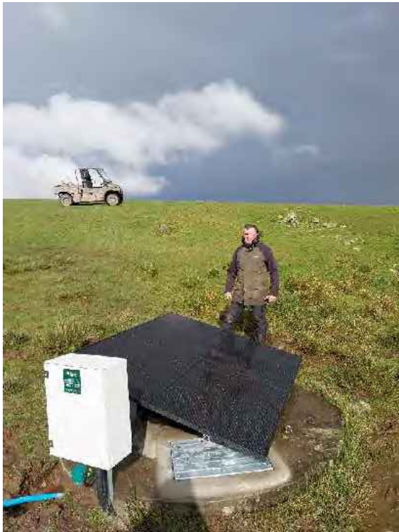
Solar powered pump for livestock watering
